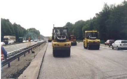
Roller positioning with total station (Geodimeter) for continuous compaction control on asphalt layers
