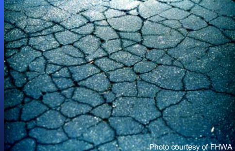
Photo courtesy of FHWA
