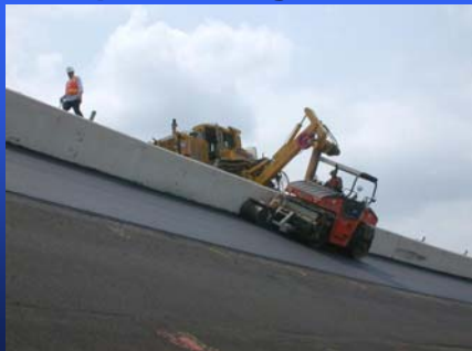
Compaction Against Wall
