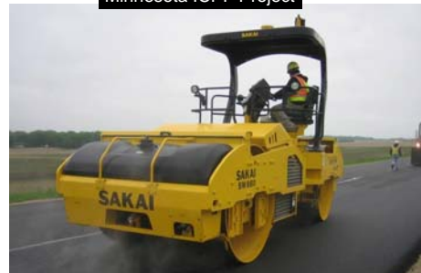
Compaction/mapping of HMA base course layer
