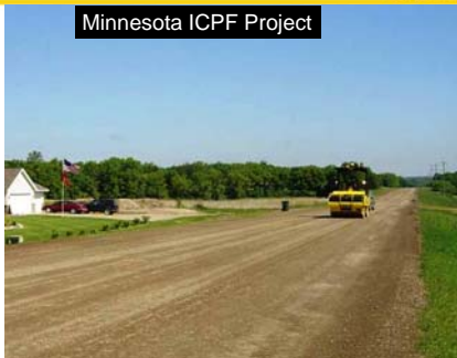
Mapping of the subgrade / agg. base layer
