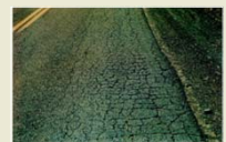
Fatigue Cracking
